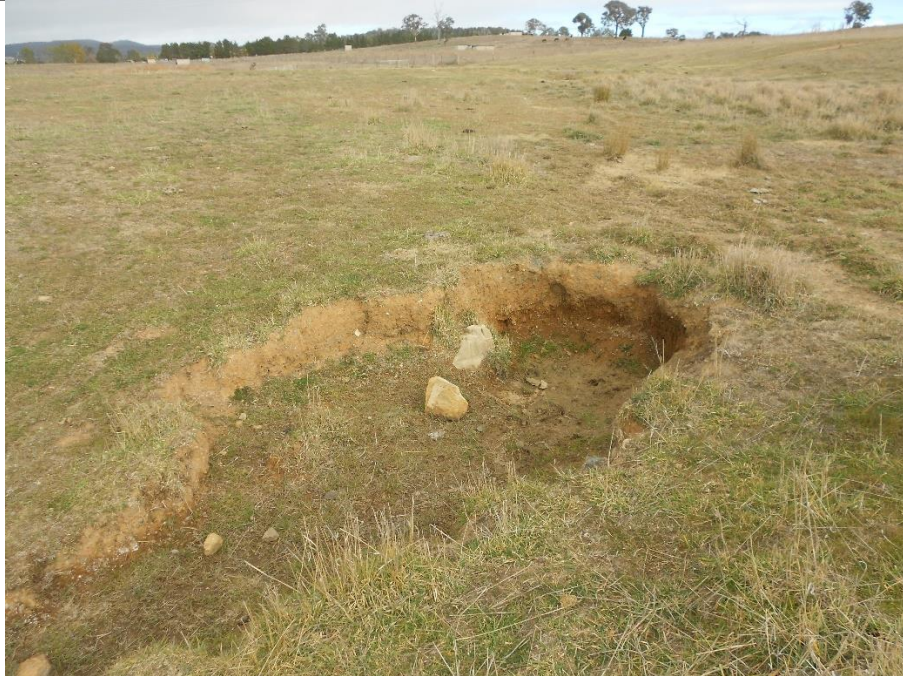
Eroding overflow of Dam 3
