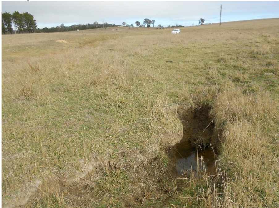
Eroding overflow of Dam 3
